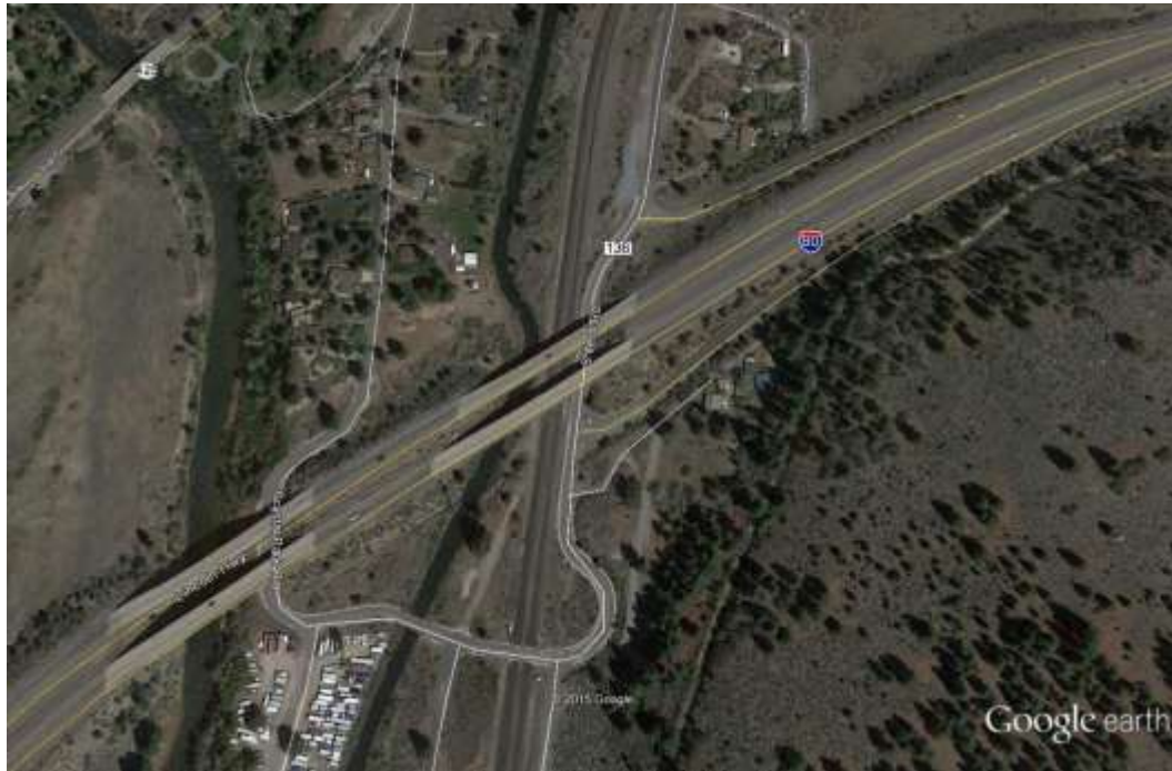
Figure 7. Google Earth view showing off- and on- ramp for Interstate 80, limited visibility to the south on South Verdi road at the off-ramp and subsequent curves prior to the rail crossing and proposed 39 Ventures site at the bottom center of the figure.
